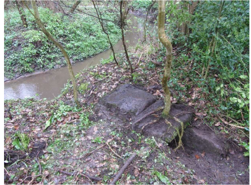
Plate X: Raby clapper bridge as seen when looking across the ditch. At the right-hand end, one of the piers may be seen protruding from beneath the slab it supports. The bridge lies in very close proximity to the river.
