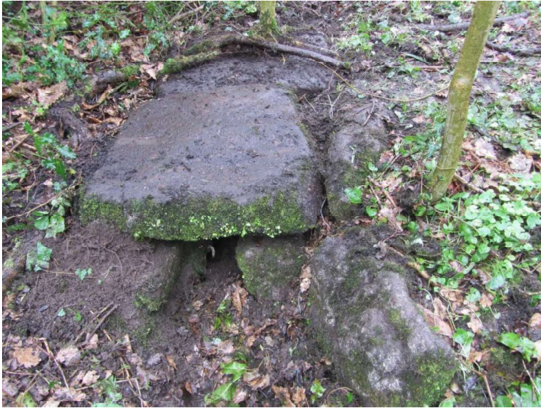
Plate IX: A front view of the Raby clapper bridge, taken looking up the ditch which it crosses. The bridge is two slabs wide, although the slab in the background is partially buried and has a tree growing upon it.
