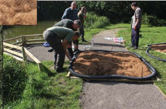
Alison fills the rafts perimeter floatation pipe with plastic bottles for extra support ( above ) Andy and David join the pipe to the wooden raft frame ( right ) The coir filled raft used to absorb algae in the pond
