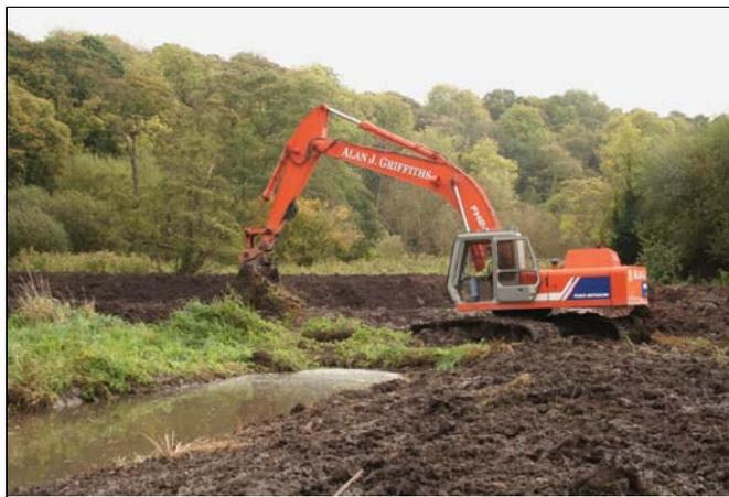
Excavator digging out pools. The dug material raising the banks for water vole burrows
